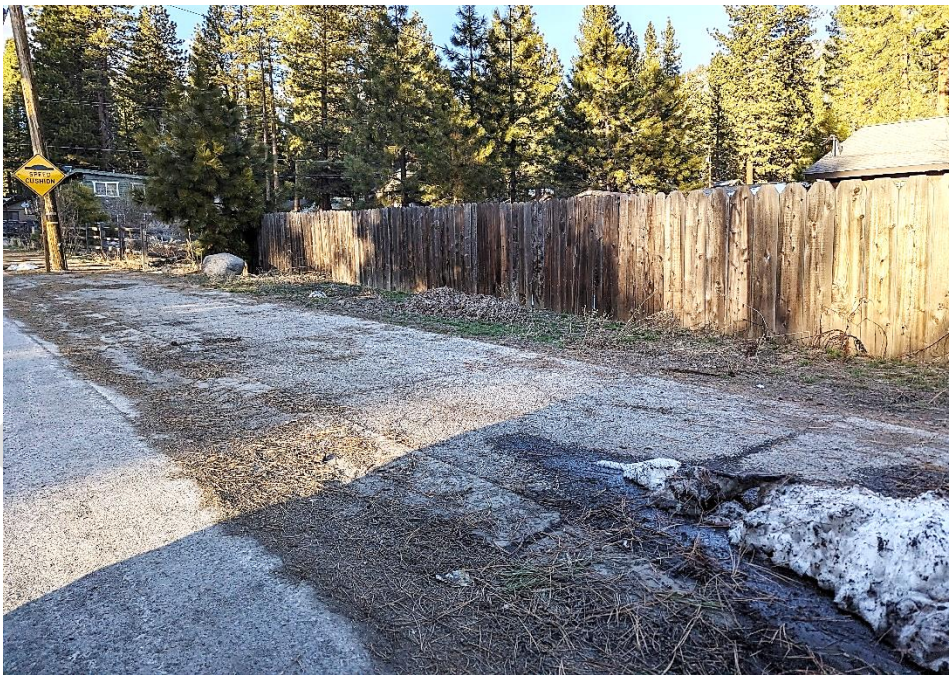
Figure 4. Pervious Parking Pad
