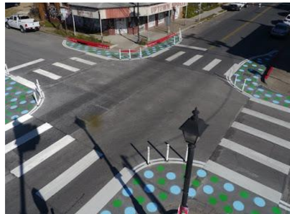
Figure 7. Temporary Intersection Curb Extension
